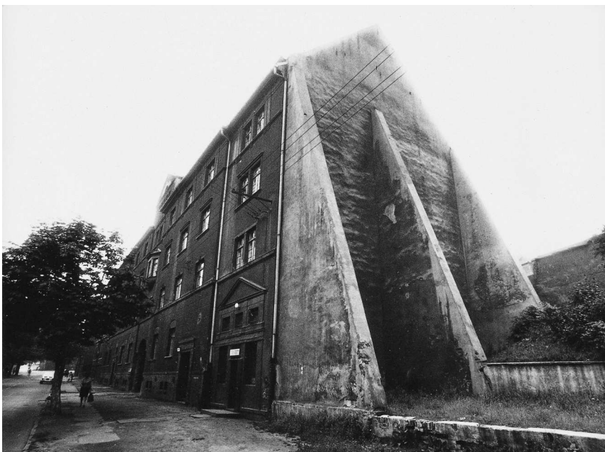
A tenement house with abutments_1978
